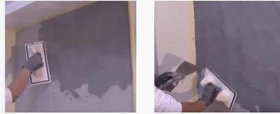
After sanding and vacuuming the second layer of Thin Microcement CimentArt, apply a third layer in the same fashion, until the surface is completely covered with Microcement.
