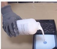
The application of the METALLIC sealer CimentArt will always be done over Thin Microcement CimentArt with a steel trowel or a sponge.
